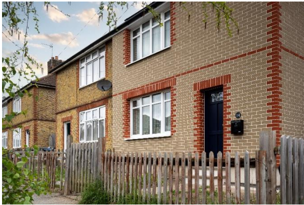
- Completed retrofitted home
